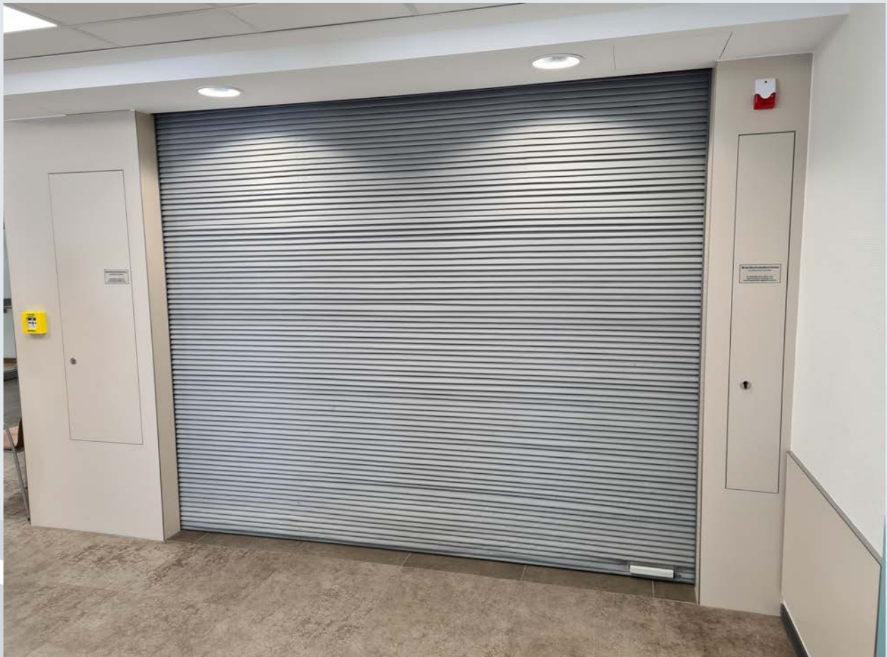
In front of elevators
